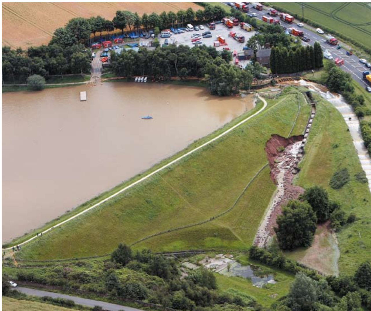
Aerial view of Ulley Reservoir after heavy rain © Empics
